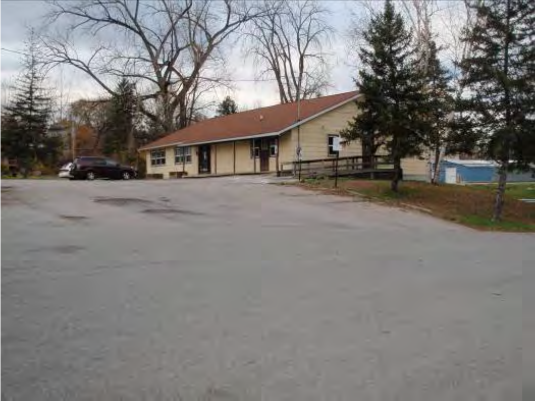
Photo 1: Former Saratoga Town Hall building, looking northeast from Route 29 (Ferry Street).
