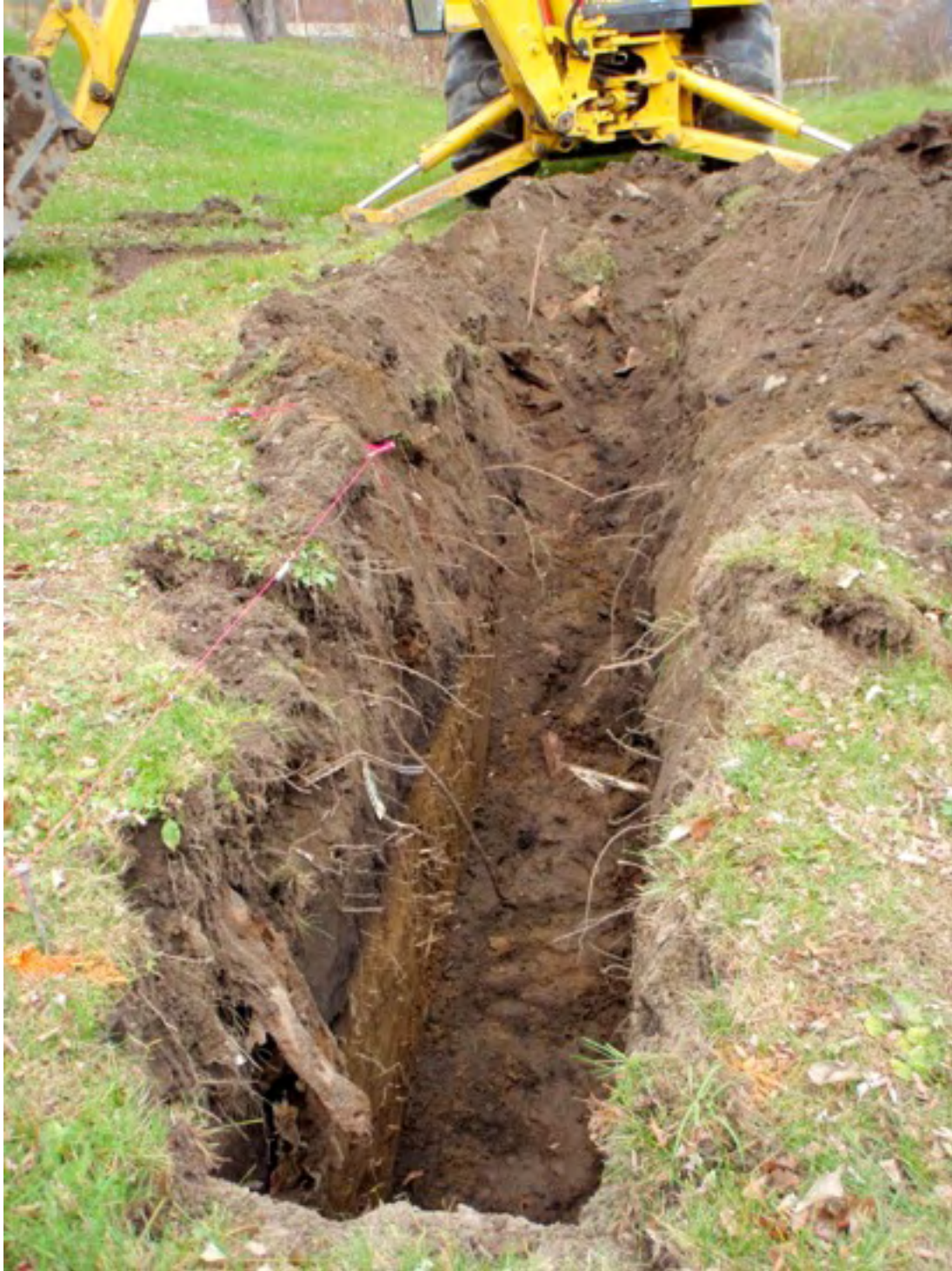
Figure 5: TR2 photo reveals dangling metal debris from the fill that buries a soil profile similar to that in TR1. TR2 was situated approximately parallel to the old Champlain Canal and just at the base of the slope leading up to the towpath road.
