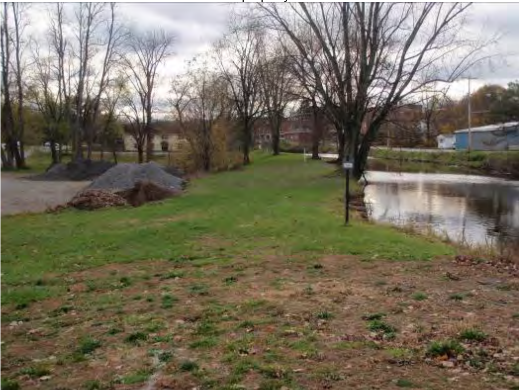
Photo 8: View looking south/southwest along the Champlain Canal towpath, with the road material area to the left, and a property line stake in the background.
