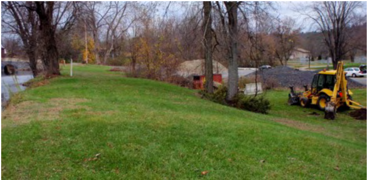
Figure 2: View northward showing the sharp elevation difference between the old Champlain Canal and towpath road versus the low lying floodplain terrace. Trench 2 location is visible at the edge of the photo.
